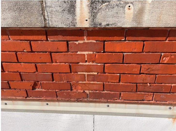
Parapet brick repair
